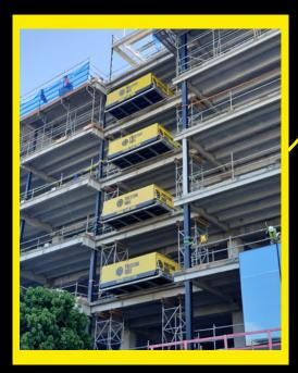
Able to be stacked vertically, SuperDecks are retractable and can be used as a drawer-like system.
