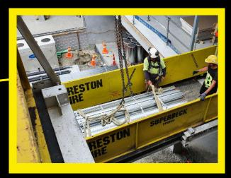
Installed vertically in as little as 15 minutes, using a two prop method or a bolt down method.
